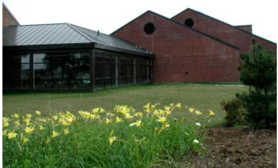
Exterior view of Cafeteria
